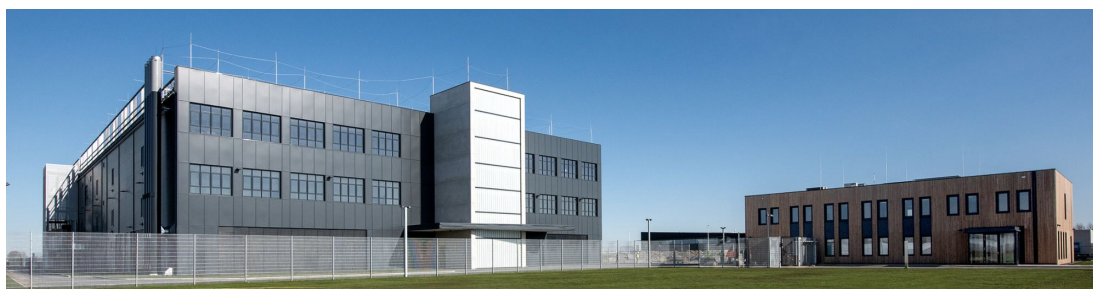
Figure 3 Amsterdam 1 data centre
